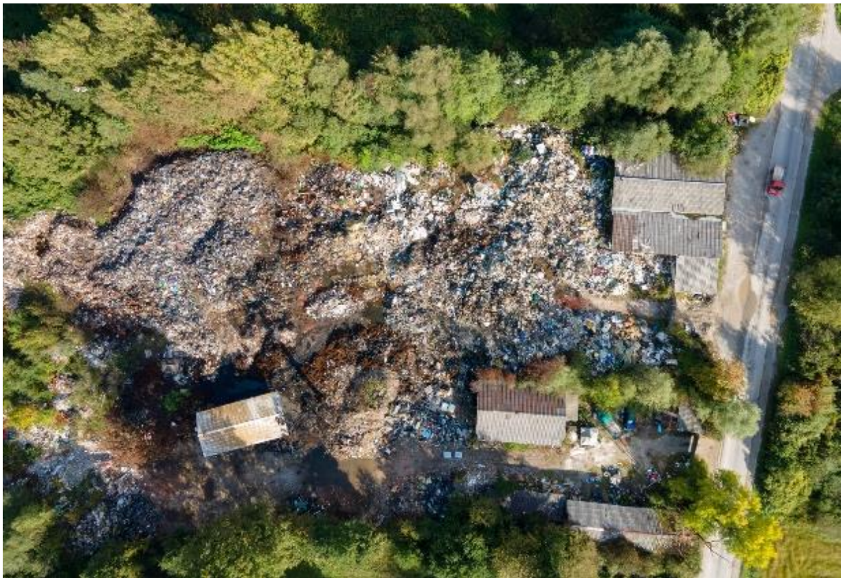
Fig 5. An example of an illegal landfill – disposal of hazardous waste in the immediate hinterland of the Slovenian capital Ljubljana (a). In August 2020, there were two major fires in the landfill area (b).
